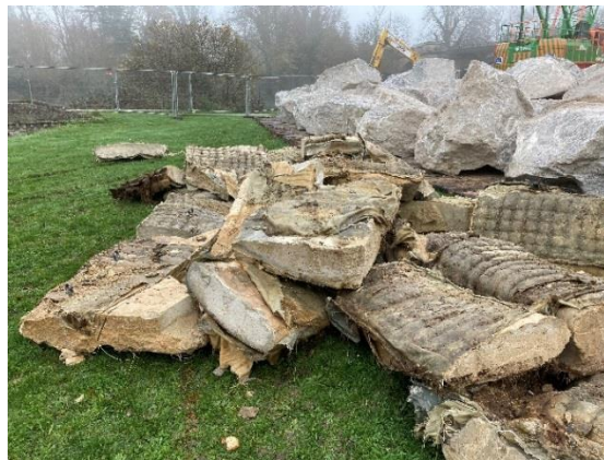
6. Removal of damaged grout mattress, with the new rock armour in the background (9 Dec)
