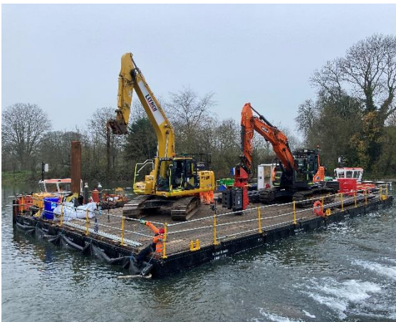
6. Removal of damaged grout mattress, with the new rock armour in the background (9 Dec)
