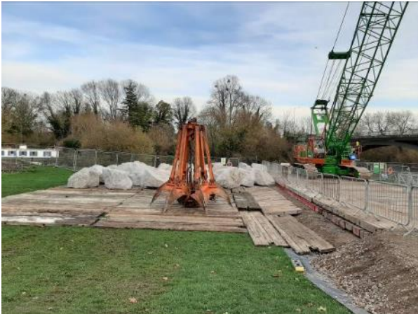
5. Cranes on floating pontoon by Black Potts Weir, operations taking place (7 Dec)
