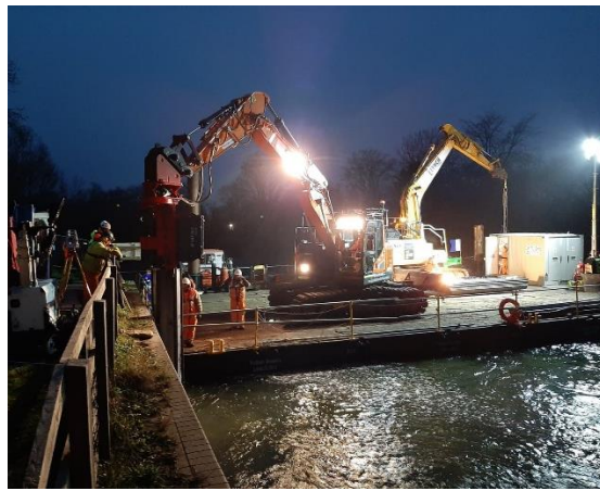
6. Removal of damaged grout mattress, with the new rock armour in the background (9 Dec)
