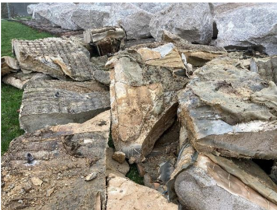
6. Removal of damaged grout mattress, with the new rock armour in the background (9 Dec)
