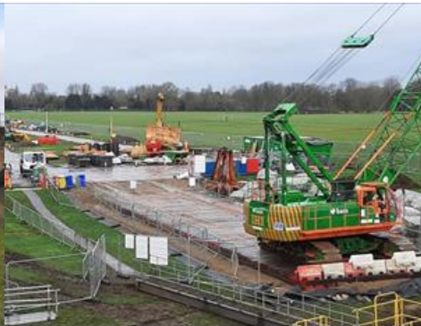
Feb 21: Site compound
