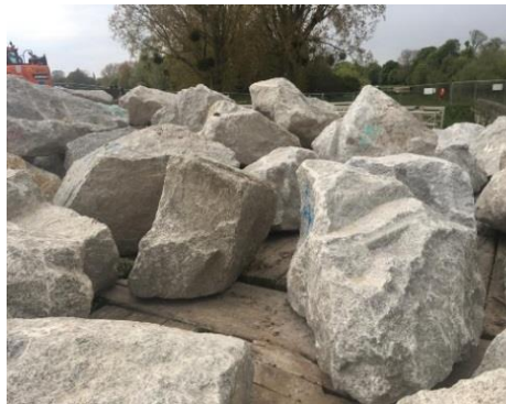
Rock armour waiting to be placed following completion of weir apron
