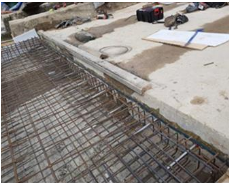
March 2021: Section of base showing the steel wire reinforcement.
