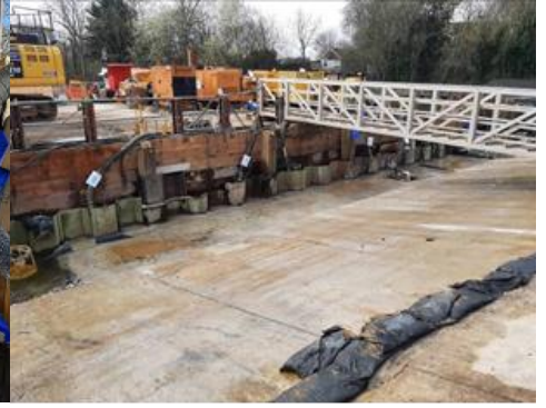
March 2021: Completed blinding
