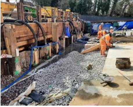
March 2021: Drainage base layer being installed
