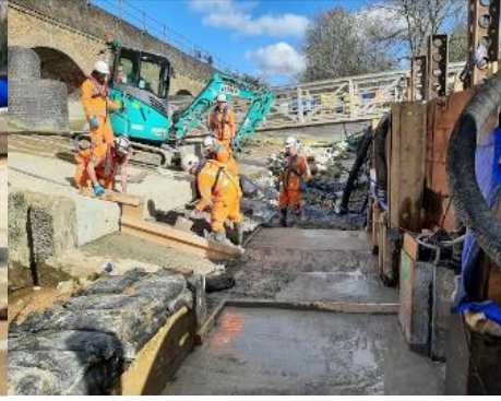
March 2021: Placing blinding layer. This is a base layer of concrete
