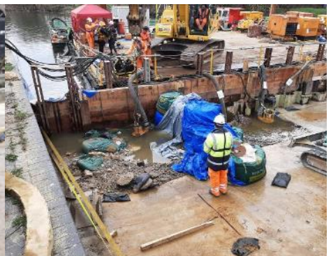
March 21: Pumping out the working area. Note wooden stop logs inserted between piles to create a cofferdam
