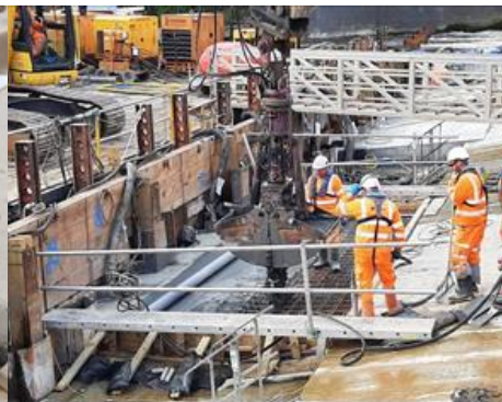
April 2021: Casting high density concrete
