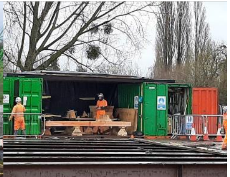
Feb 21: Preparing stop logs whilst we were unable to work in the water during high flows
