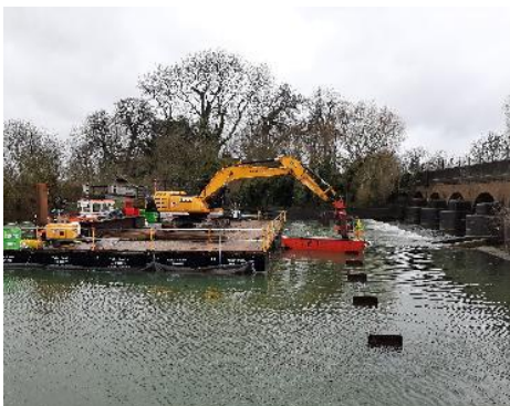
Feb 21: Installing piles for stop logs to slot into
