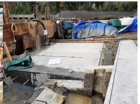
April 2021: Completed section of weir apron
