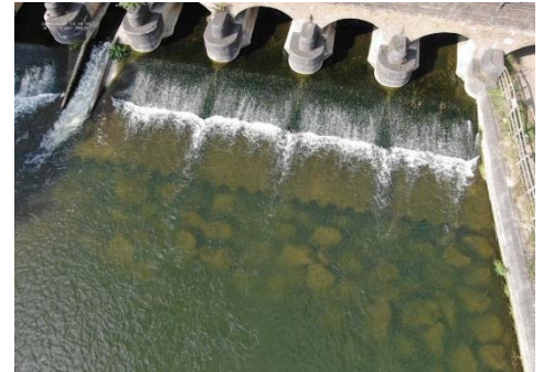
Aerial view of completed weir repairs
