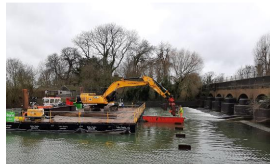
Installing sheet piles
